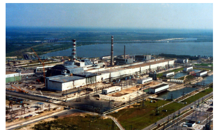
Chernobyl Nuclear Power Plant
