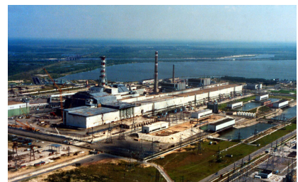
Chernobyl Nuclear Power Plant
